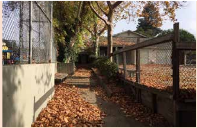
CDC Building January 2021
